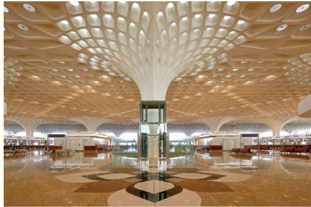
Chhatrapati Shivaji International Airport Terminal 2, Mumbai
